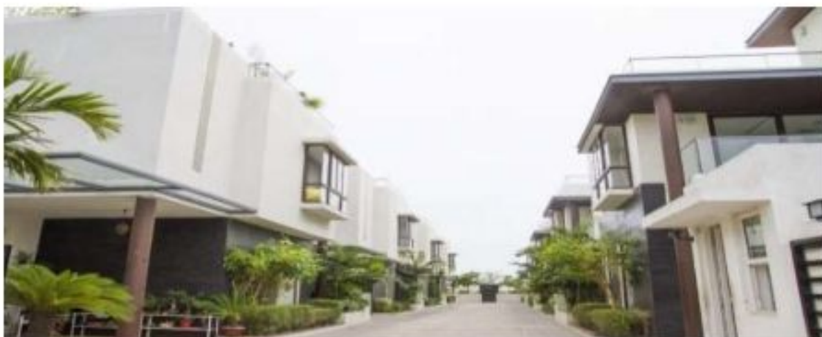
Houses in Gated Community as Per Building Bye Laws Regulations
