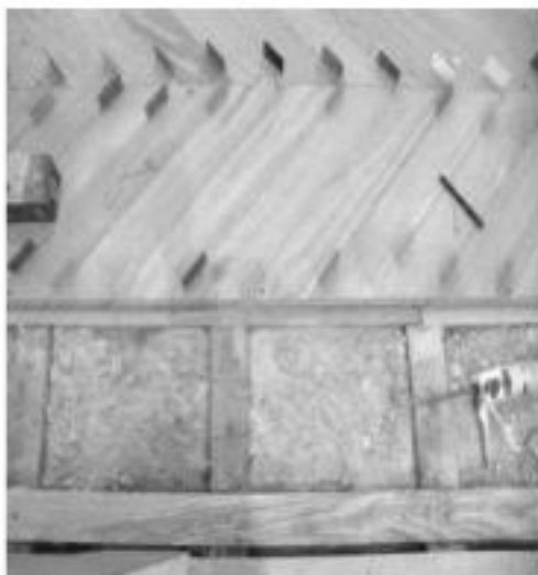
Figure 18. Application of solid wood parquet
