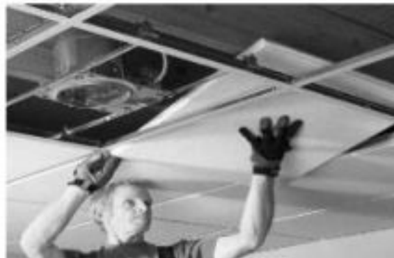
Figure 4: Installation of suspended ceiling
