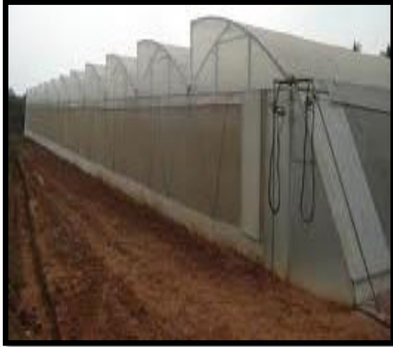
Poly-house Structure for Nursery
